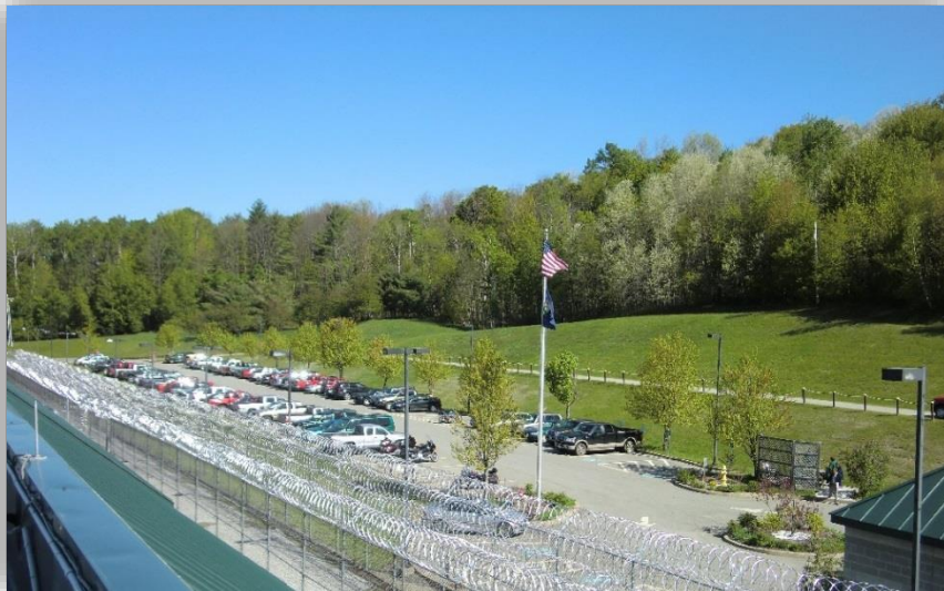
EXISTING PARKING LOT AND PERIMETER ROAD
