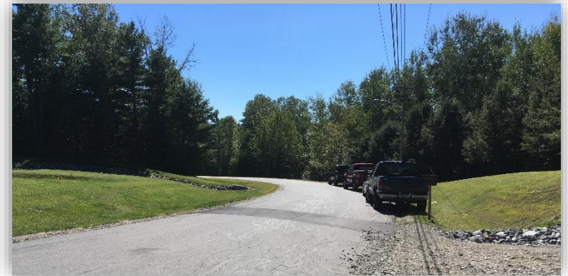
TYPICAL OVERFLOW PARKING CONDITIONS
